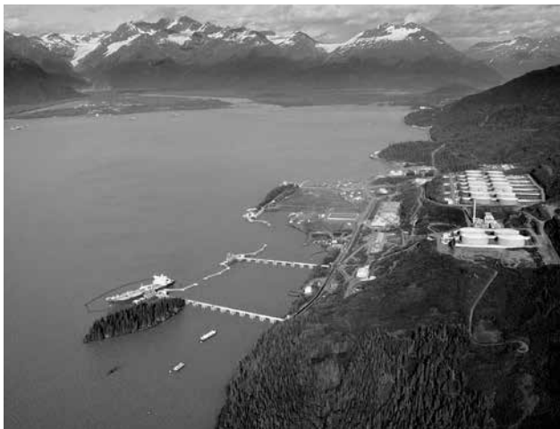
Valdez Marine Terminal (VMT).
