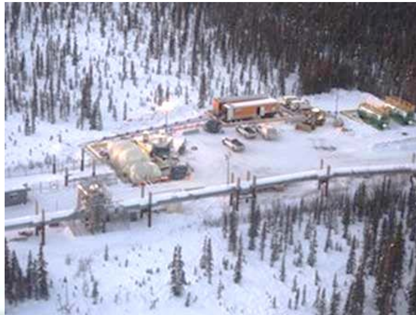
Slip Stream Heat Operation
